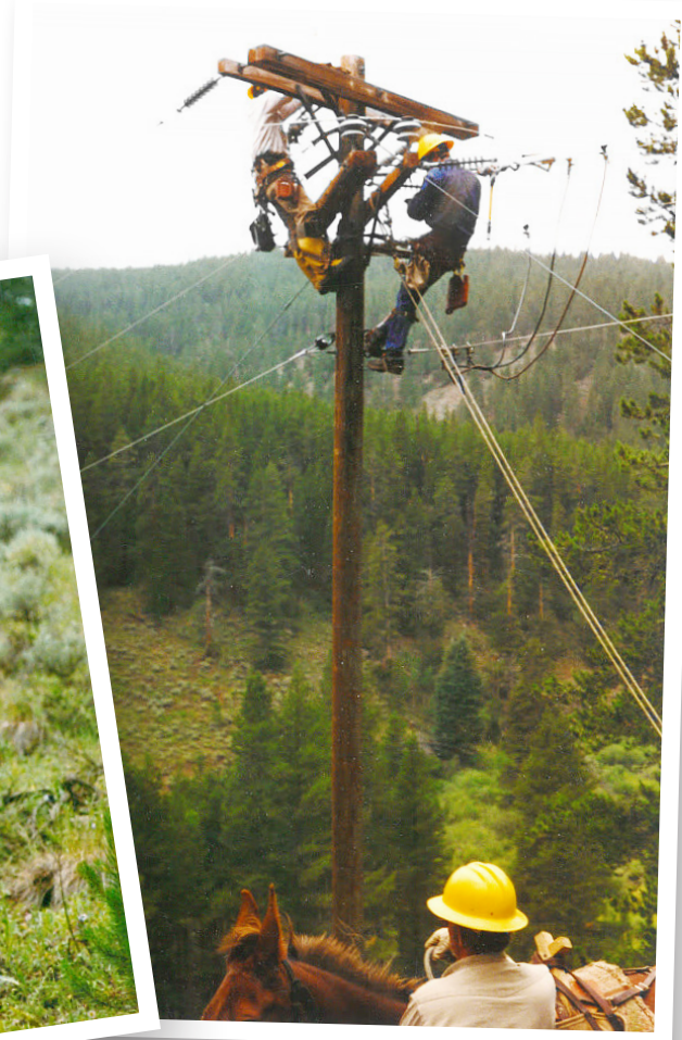
(Below) Marc Karo and Nathan Klindt changing burned-out insulator bells while John Purdue and Sheila look on.
