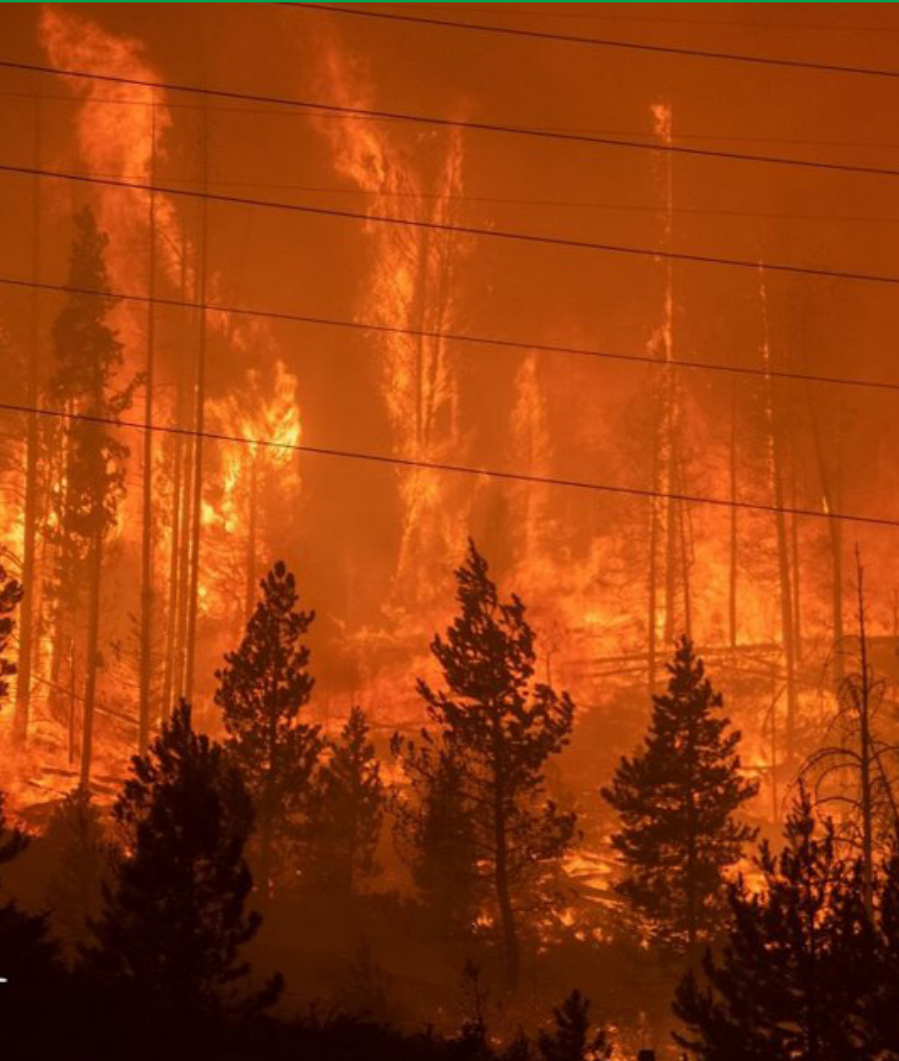
The East Troublesome Fire destroyed miles of MPE's overhead lines.
