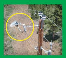
A broken porcelain cutout was photographed on Ten Creek Road east of Granby by a SAM drone pilot, recognized by a SAM inspector, and sent immediately on July 16 to the Operations Department at MPE.
