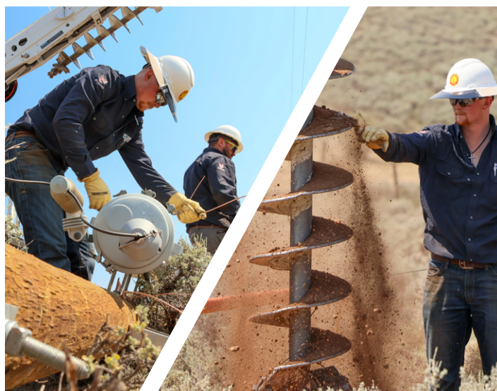
John Butler in his second week as a summer intern with the Kremmling line crew helped to complete a pole change-out near Williams Fork Reservoir.
